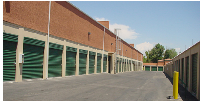
Completed Project: Mini-Storage @ Jones & University
