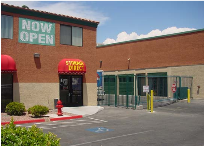
Completed Project: Mini-Storage @ Jones & University
