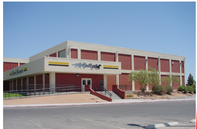
Southwest Exterior Façade of the Auxiliary Gymnasium at Clark High School, Las Vegas, Nevada
